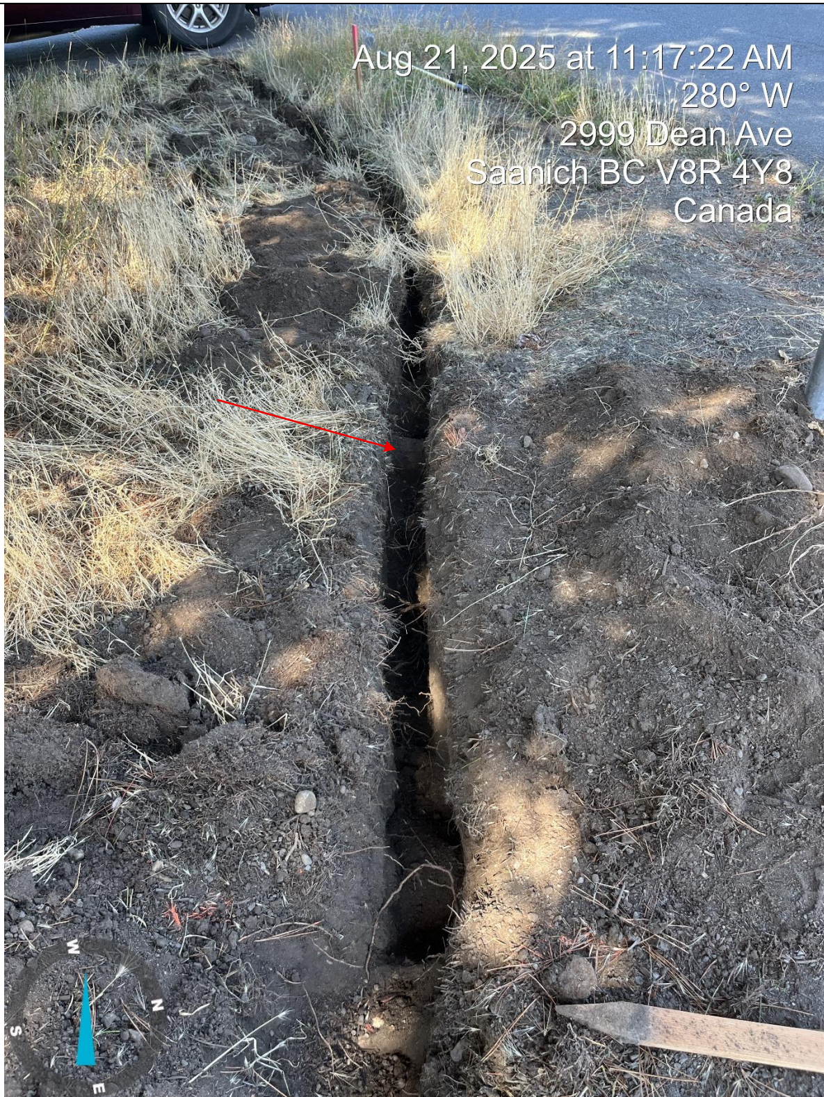
Photograph 5: Area of hand-dug exploratory excavation along the backside of the proposed sidewalk (wooden stake – red arrow) on the north side of tree 2249. The large ~12-14cm root exposed .25m from the existing stop sign can be seen (blue arrow).
