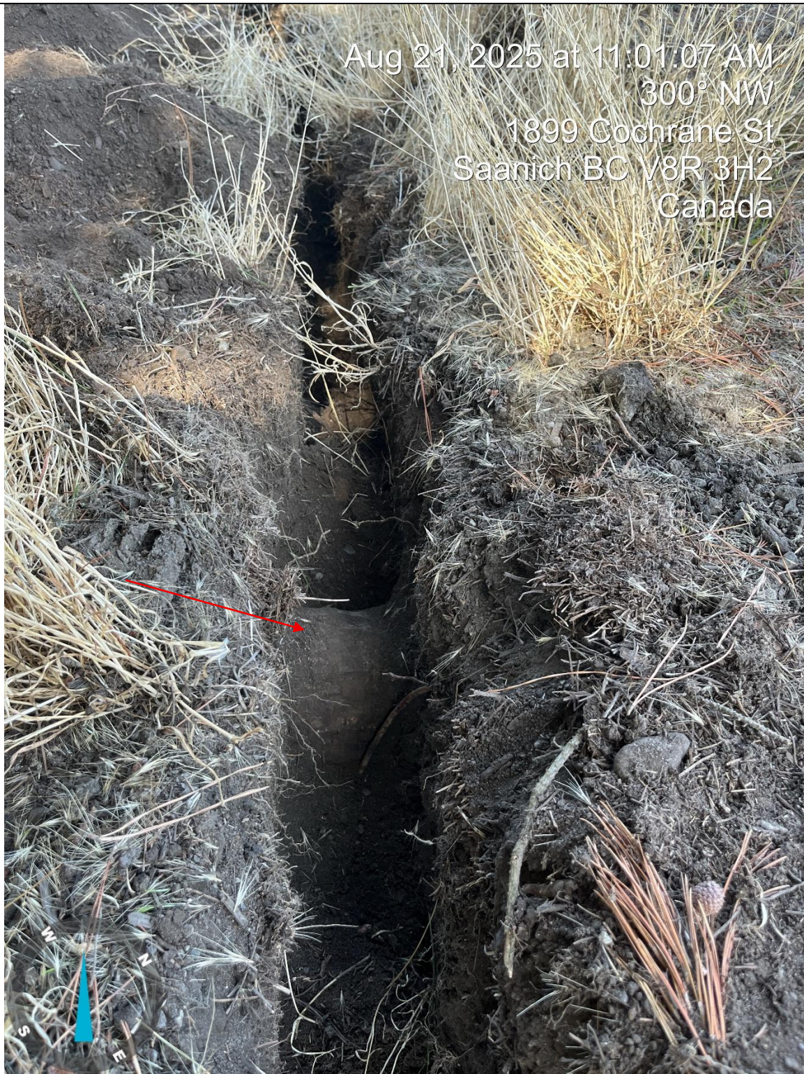
Photograph 4: Area of hand-dug exploratory excavation along the backside of the proposed sidewalk on the north side of tree 2249. Large ~12-14cm root (red arrow) was exposed roughly .25m west from the existing stop sign at the corner of Cochrane Street and Dean Avenue.
