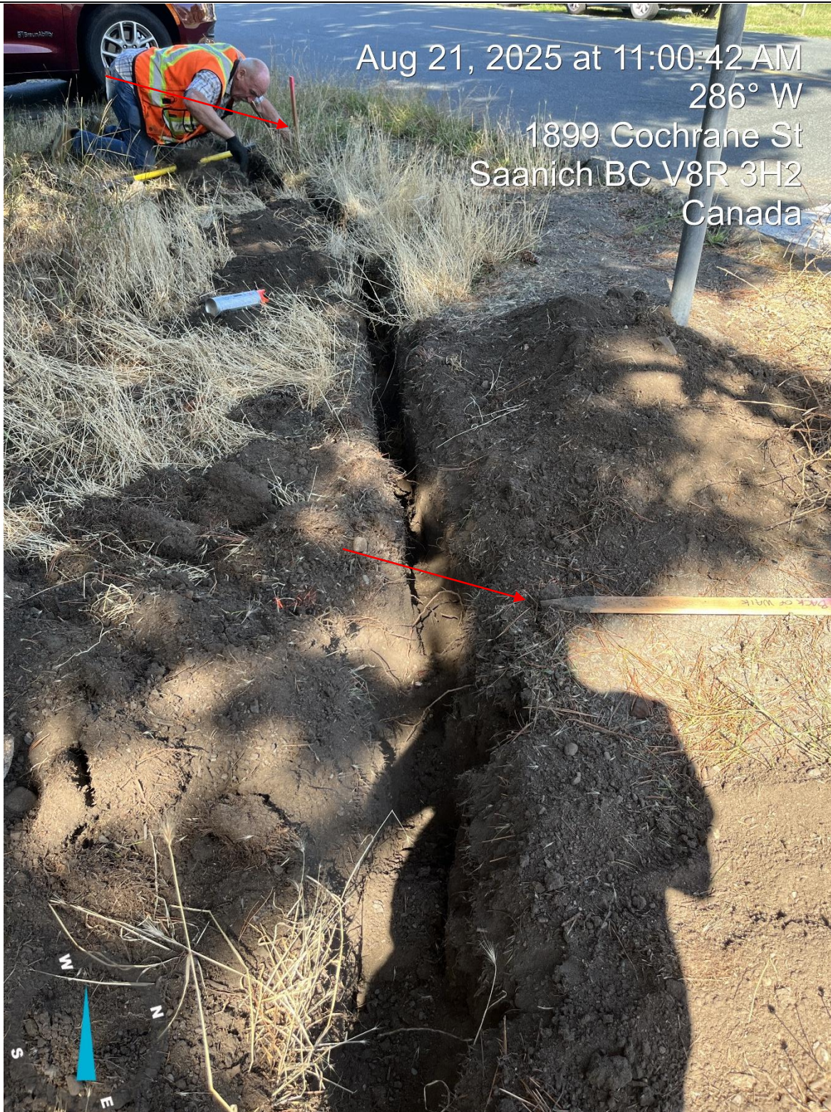
Photograph 3: Area of hand-dug exploratory excavation along the backside of the proposed sidewalk (wooden stake – red arrow) on the north/northeastern side of tree 2249.
