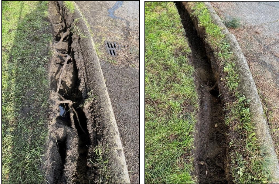
Photographs 1 & 2: Larger rooting structures (~10-20cm in diameter) were exposed approximately 5-6.5m east of tree 2249 near the existing catch basin on Dean Avenue ( left photo ). More larger rooting structures encountered ~5-6m northeast from the root collar of tree 2249 ( right photo ).
